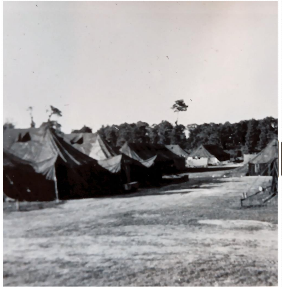
1200 bed tented hospital in Bayeaux
